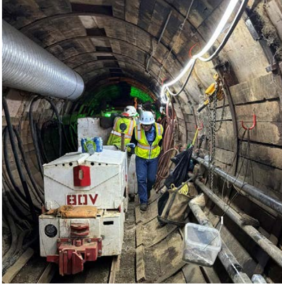
Figure 2. Images of filtration plant and pipeline construction
