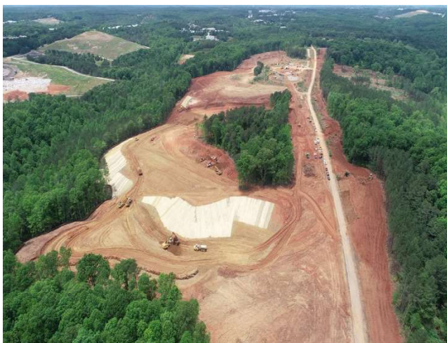
85 Business Park Construction
